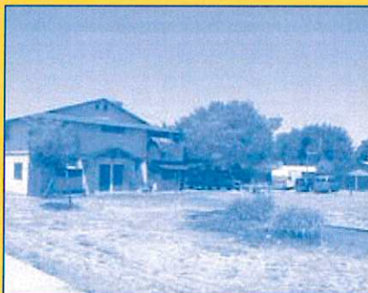
Poorly maintained property
