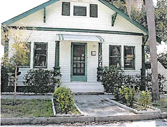
Properly selected, installed and maintained landscaping allows for unobstructed views of otherwise vulnerable doors and windows
